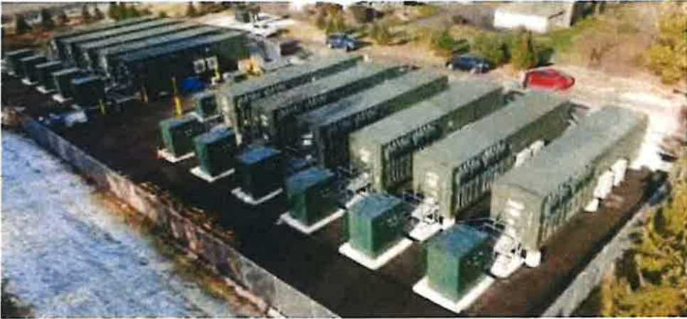
BESS Installed in Dedicated Structure
