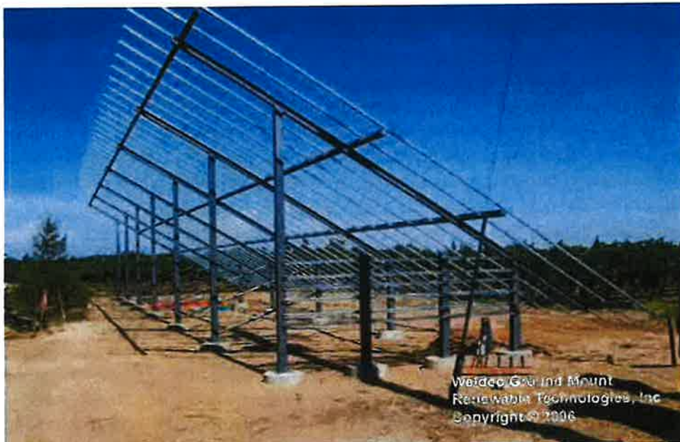
Typical fixed-tilt mounting structure
