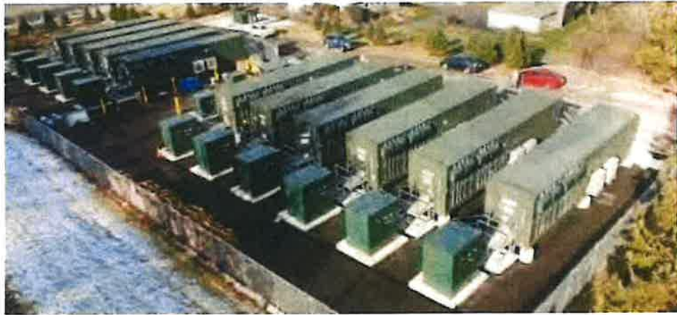
BESS Installed in Dedicated Structure
