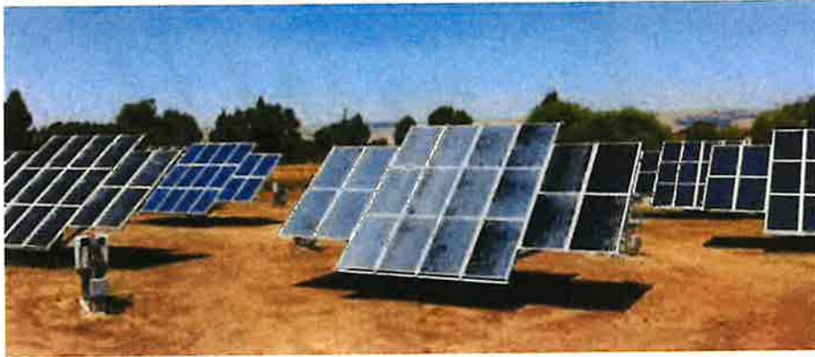
Typical dual axis tracking solar panels
