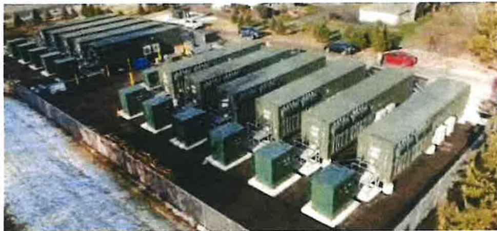
BESS Installed in Dedicated Structure
