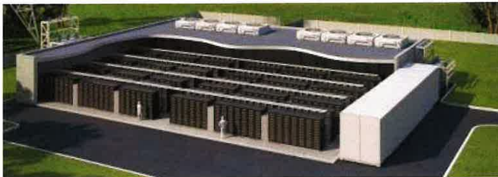
BESS Installed in Dedicated Structure
