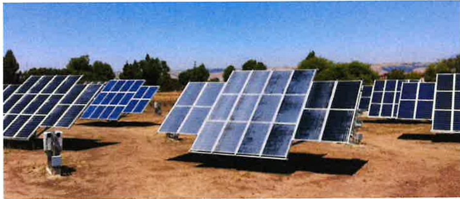
Typical dual axis tracking solar panels
