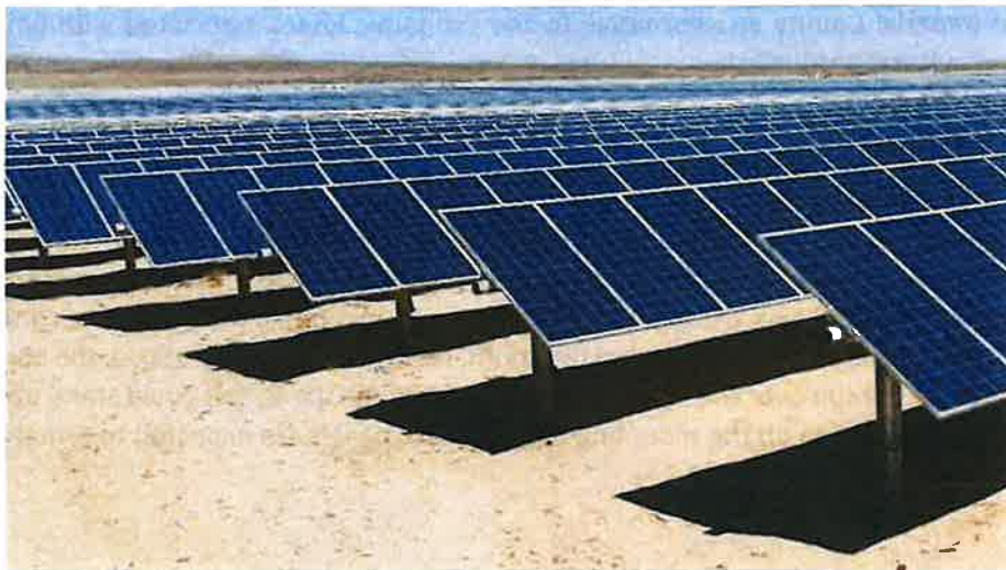
Typical single axis tracking solar panels
