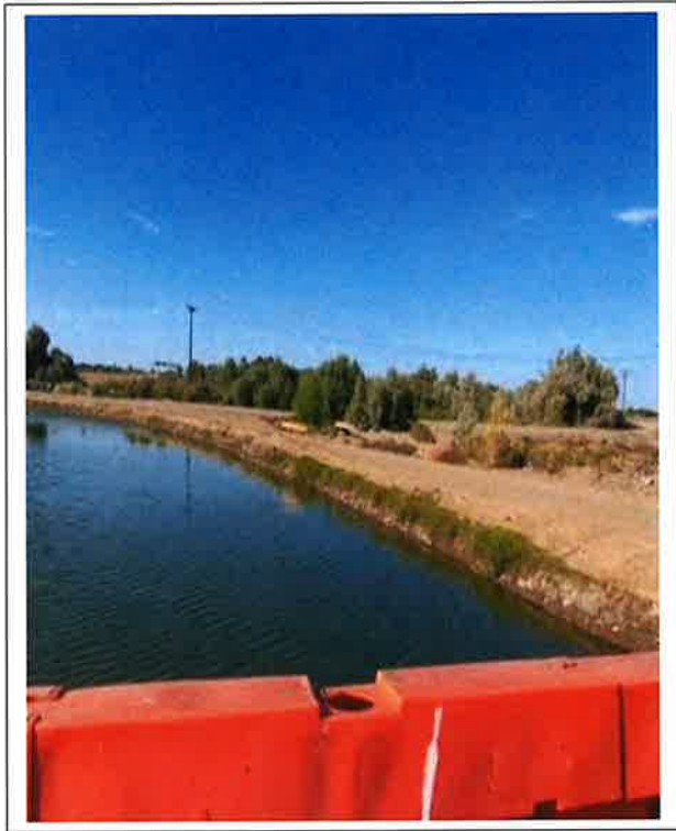
5. Facing south while on bridge 8/8
