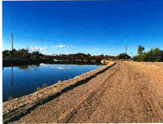
Figure 7: Overview of Yuma Main Canal and Picacho Bridge access road, view to the south-southeast
