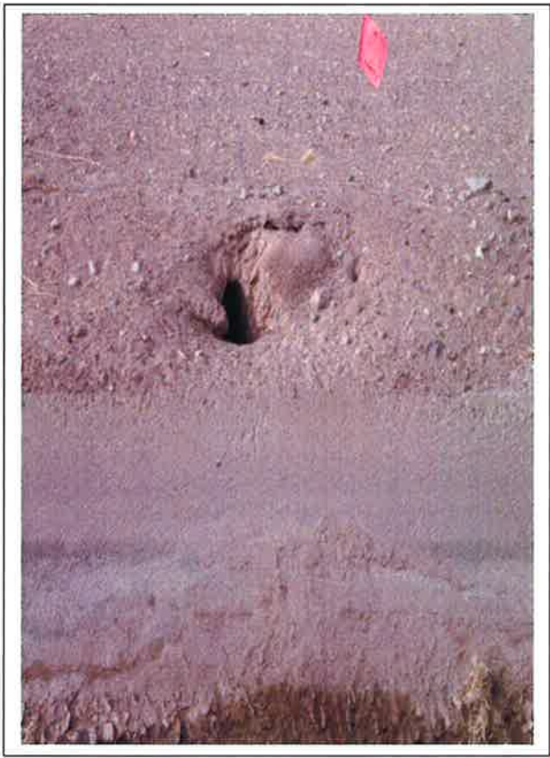
9. Active burrow along Nectarine Lateral A canal offsite to the south of site
