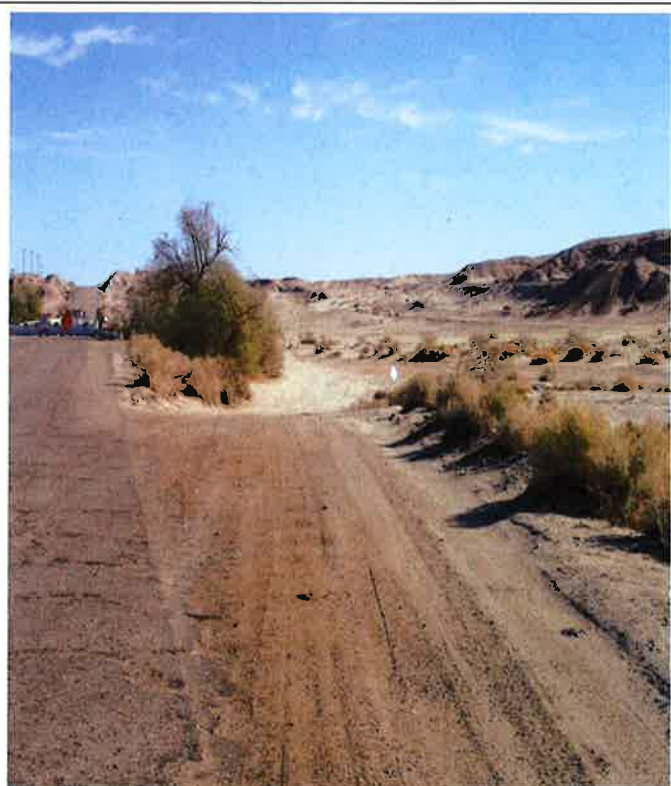
9. Illegal bypass road around bridge looking east
