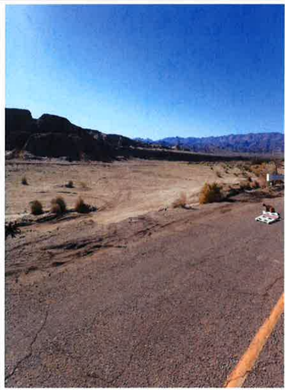
4. Area to south of bridge; area being used illegally as a bypass to closed bridge
