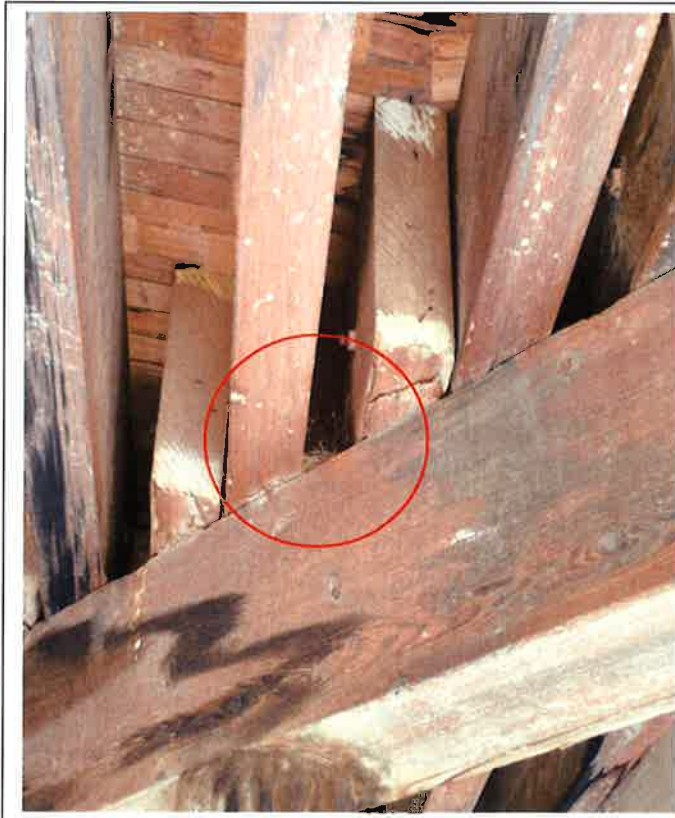
13. Abandoned nest in bridge supports
