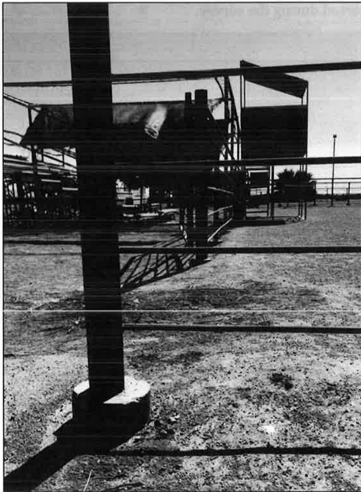
Close up of arena and concrete footings.
