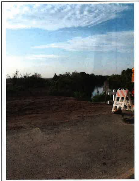
6. North side of river on Lack Rd. looking east.
