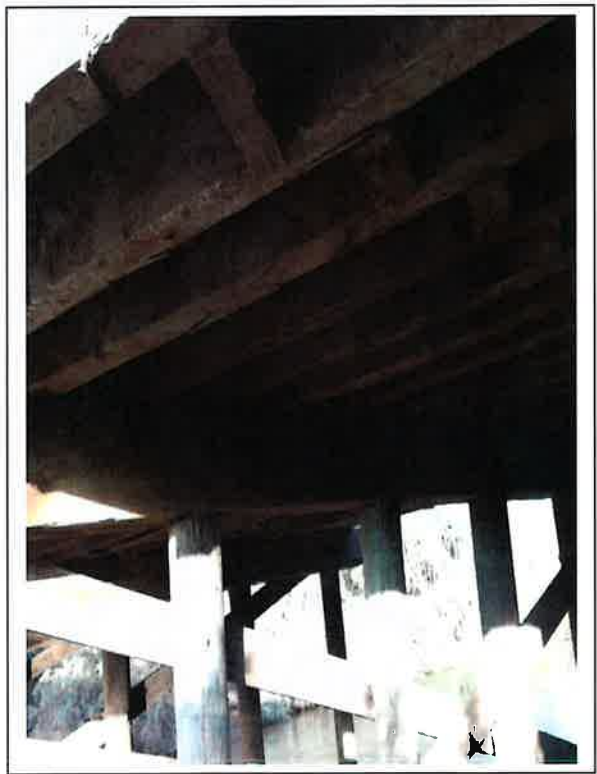
8. From the south Bank of the New River the picture taken is from the midsection of the bridge looking south, no nesting birds or bats were observed.
