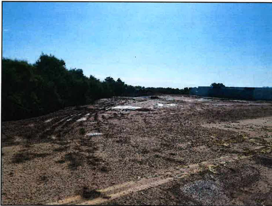
EXHIBIT 3: OVERVIEW OF API/STAGING AREA, VIEW NORTHWEST.
