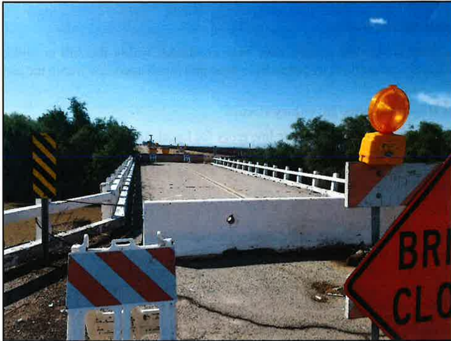
EXHIBIT 4: OVERVIEW OF EXISTING BRIDGE, VIEW SOUTH.
