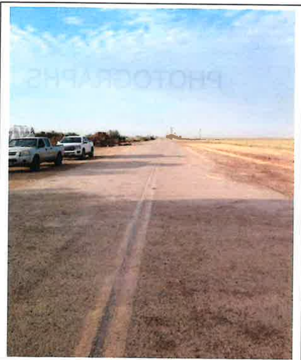
3. South end of the New River bridge looking south on Lack Rd.
