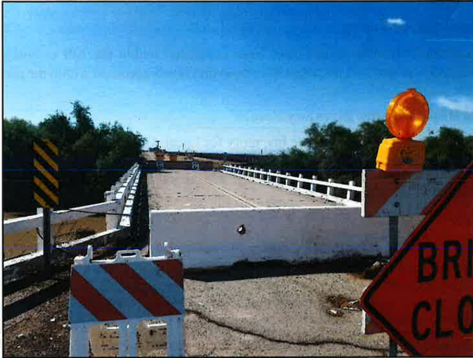
EXHIBIT 4: OVERVIEW OF EXISTING BRIDGE, VIEW SOUTH.
