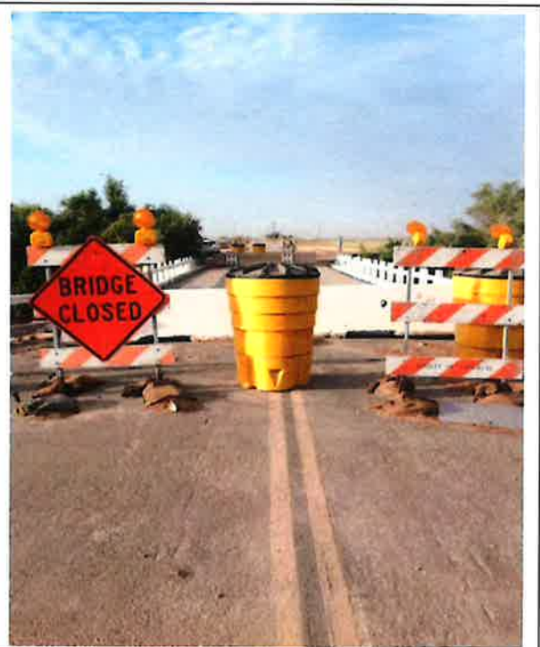
4. On Lack Rd. looking south across the New River Bridge.
