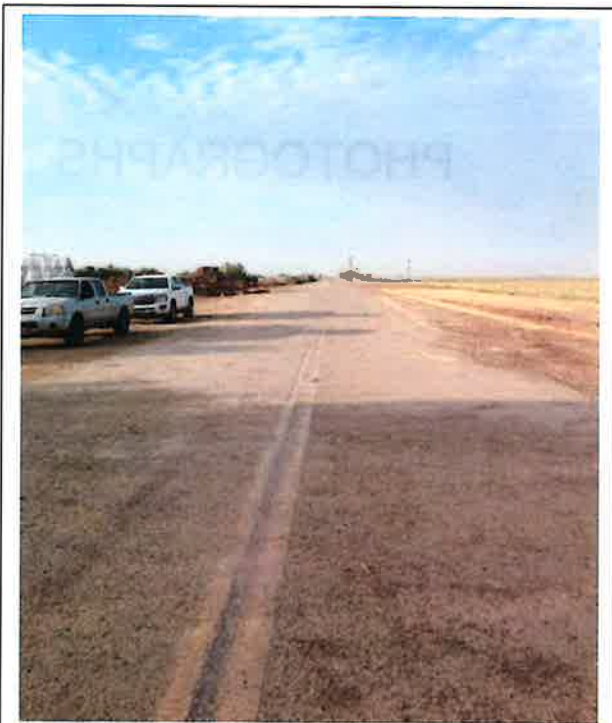
3. South end of the New River bridge looking south on Lack Rd.
