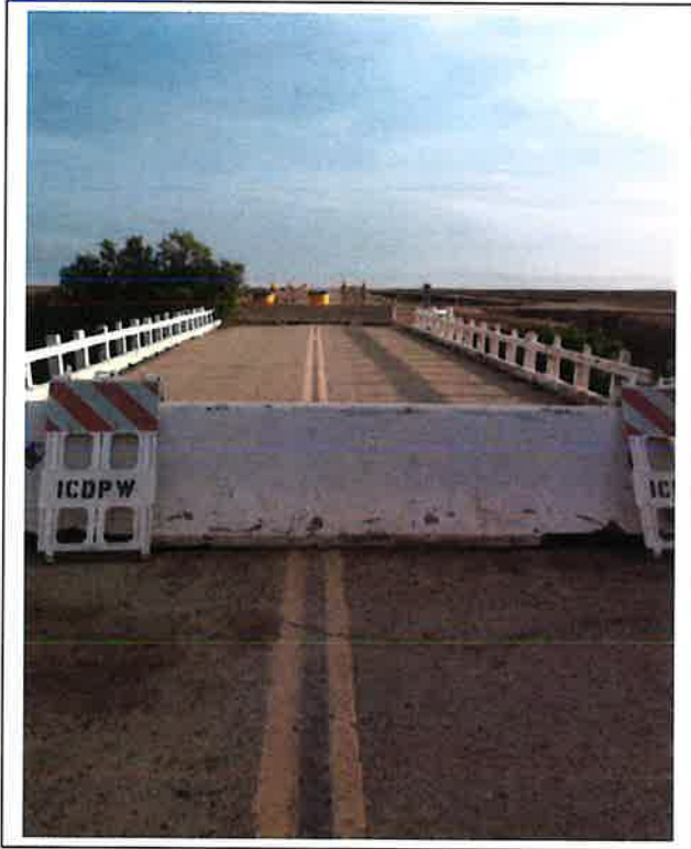
1. New River bridge on Lack Rd. looking north.
