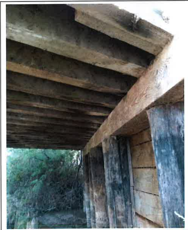
7. Under the bridge on the north bank no nesting birds or bats were observed.
